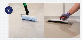
Application of **GRIP A936 XPRESS** (100g/m²) on the resin and after 2h apply the self-levelling compound over the entire surface.
