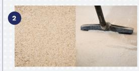
Broadcast sand (BOSTIK S409) in excess on the 2nd layer over the fresh resin, then vacuum the excess sand after 24h.
