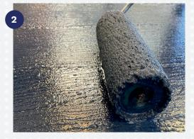
Apply the 1st coat of the undiluted HYTEC A370 RAPID using a medium hair roller at a rate of 150g/m²/coat.
