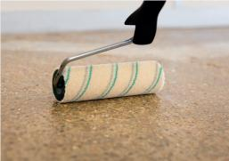
Apply with a **short hair roller** and ensure that the entire surface has been properly covered with a **continuous film**.
