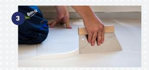
**Application of the adhesive** for soft floor covering installation.
