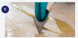
Application with a **notched trowel TKB-B2** in 2 coats at 24h intervals at a rate of 400g/m² for the 1st coat and 300g/m² for the 2nd coat.
