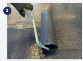
After **30 minutes of drying,** apply the **2nd coat** perpendicularly and allow to **dry for about 1-2h.**
