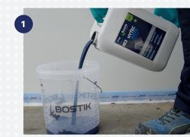
Pour HYTEC A370 RAPID into a **clean bucket or paint tray to facilitate** the application of the medium hair roller.
